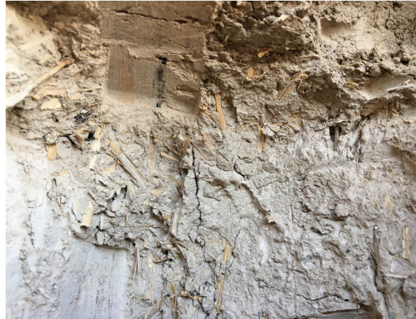
06a and b Uruk, Eanna Ziggurat west corner before conservation work (a) and yellow straw in the mortar of the existing fabric (b)
