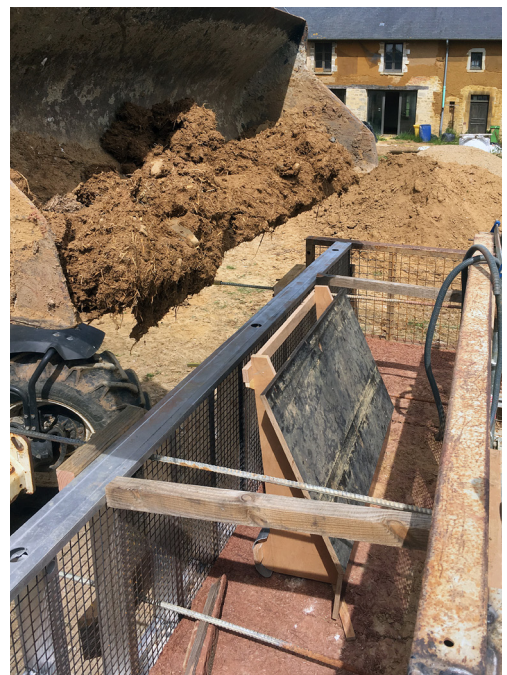
11 Intermediate formwork designed for filling material from a digger bucket
