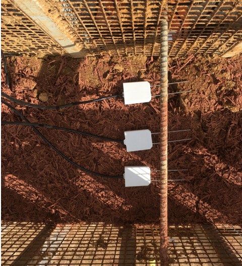
12 Installation of sensor probes for measuring water humidity and heat transfer
