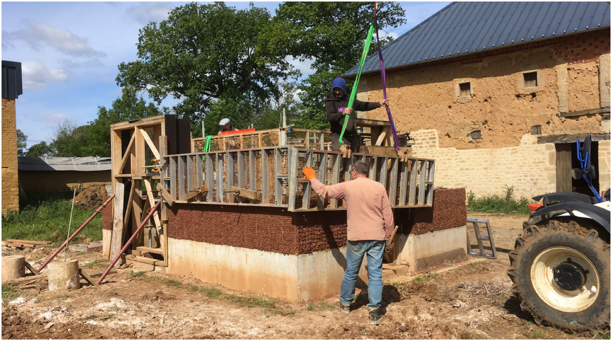
09 Aligning two mesh formwork panels for the next lift
