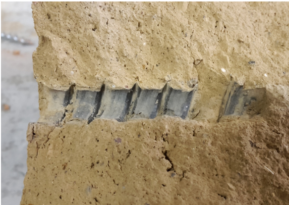
Anchor channel in earth block
