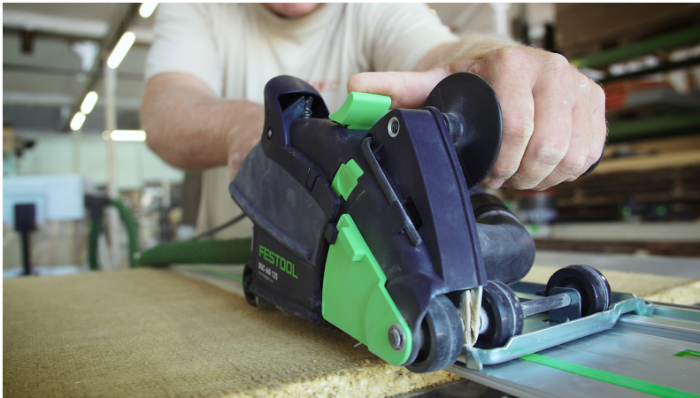
Cutting of earth drywall board using the FESTOOL separation system
