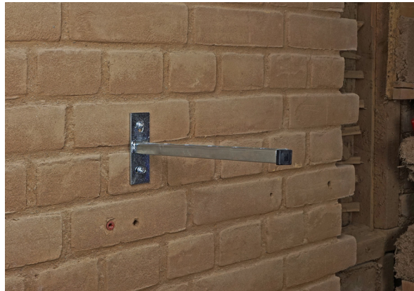
Supporting bracket in earth brick wall
