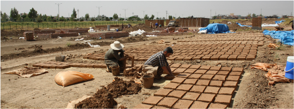
09 Building site: Production of earth blocks
