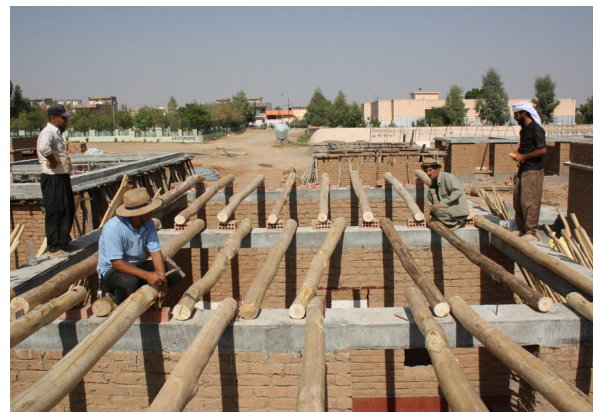
11 Building site: The roof
