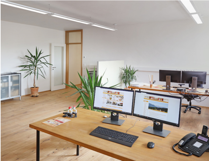
02 The heating and cooling climate panels in the office ensure pleasant working conditions all year round
