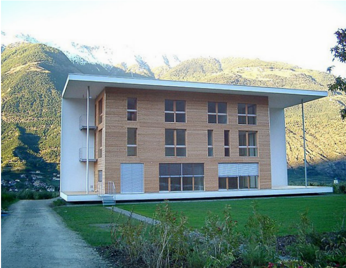
09 Modern house in north Italy (2012) – for summer cooling, the water for the climate panels passes through a ground collector
