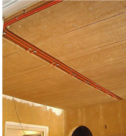
10 Ceiling-mounted WEM climate panels in a modern timber house in northern Italy (2005)
