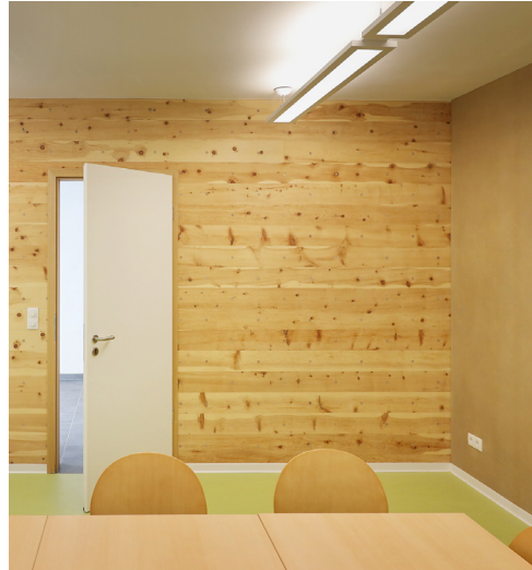
03 WEM climate panel ceiling made of earth for heating and cooling combined with Holz100 timber walling in the conference room.
