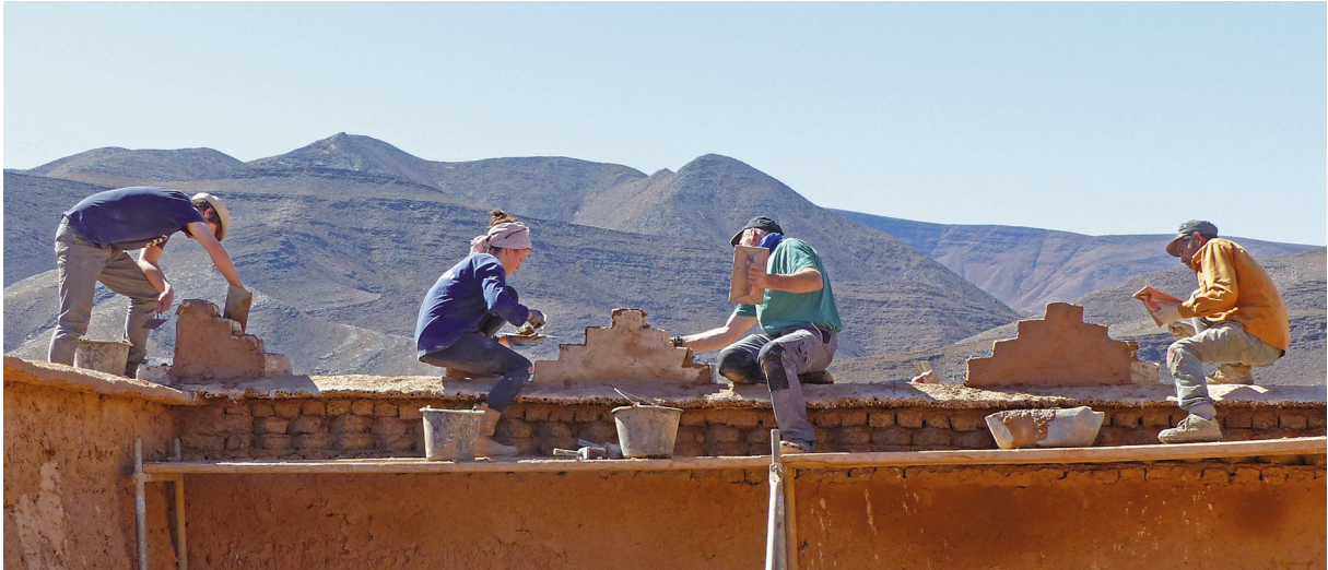
02 Plastering the “crenelations” with a fine-grain lime-earth plaster, Kasbah des Caid, Tamnougalt, Morocco
