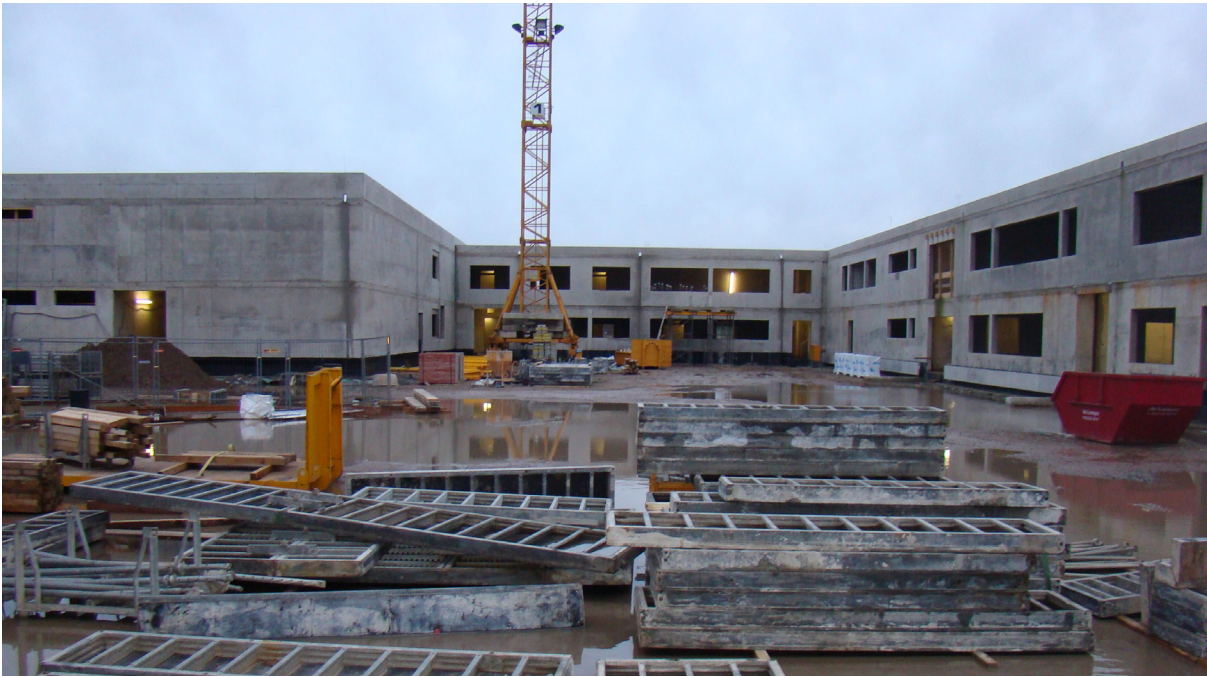
02 The new office building during construction. The find depot (left) is clearly recognisable due to its lack of windows
