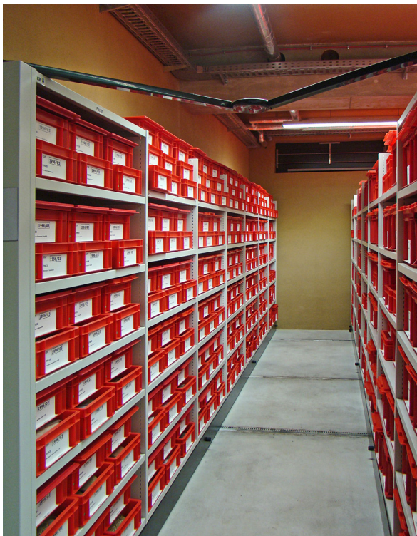
05 Sliding shelf system with red boxes containing finds showing clay plaster walls and smoke extraction vents
